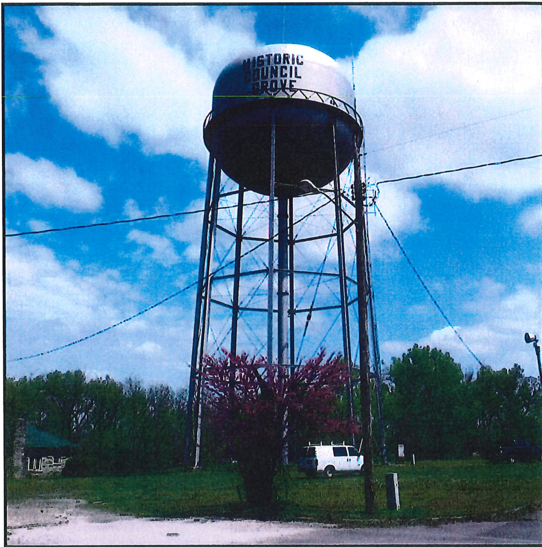
Tank Size and Style: 500,000 Gallon Double Ellipsoidal
