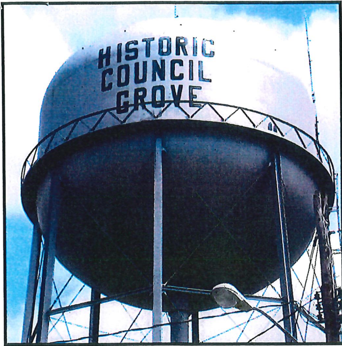
Overall view of tank exterior.
